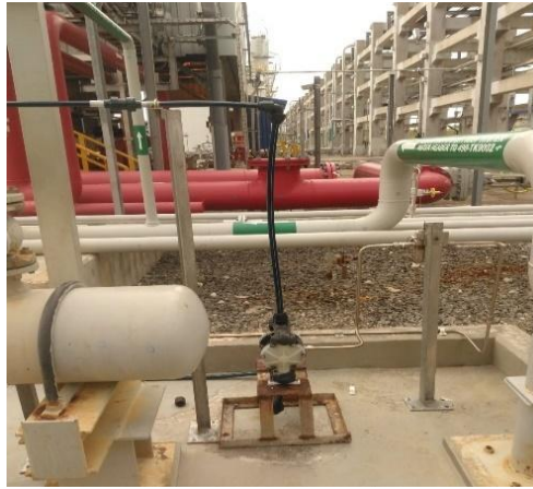
Gambar 3. Air Operated Double Diaphragm (AODD) Pump
